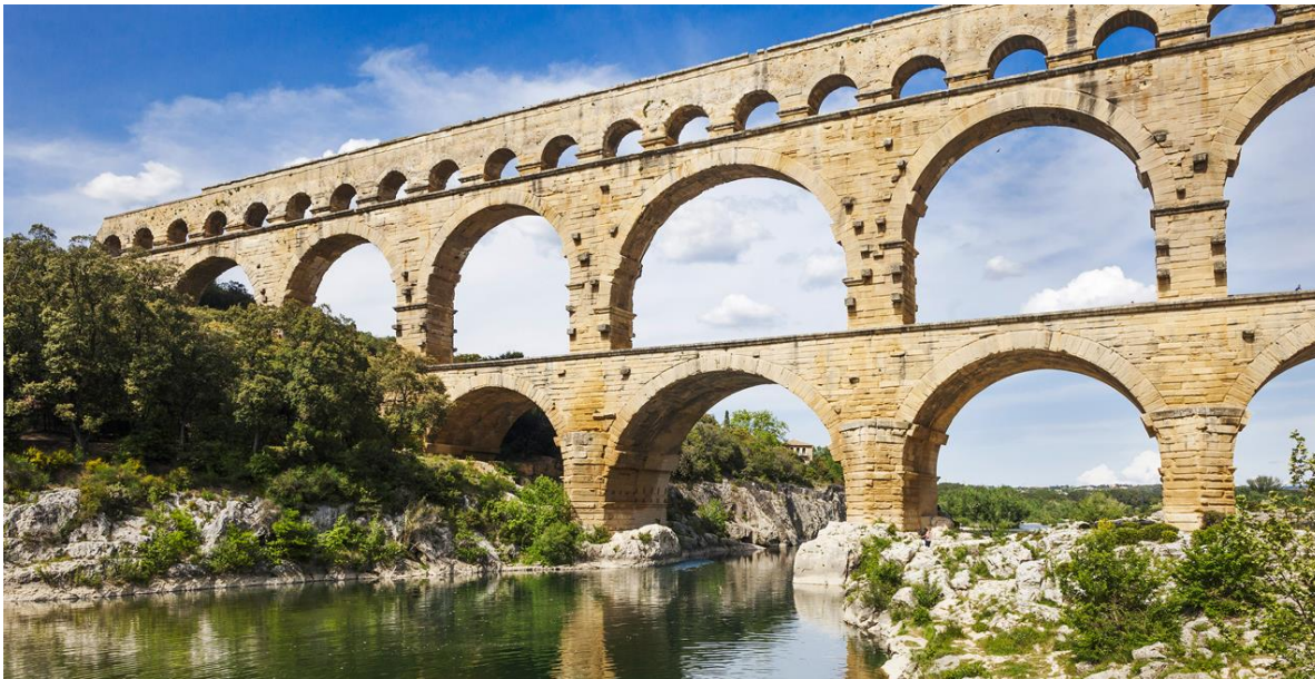
Bridge of the Gard (F)...
